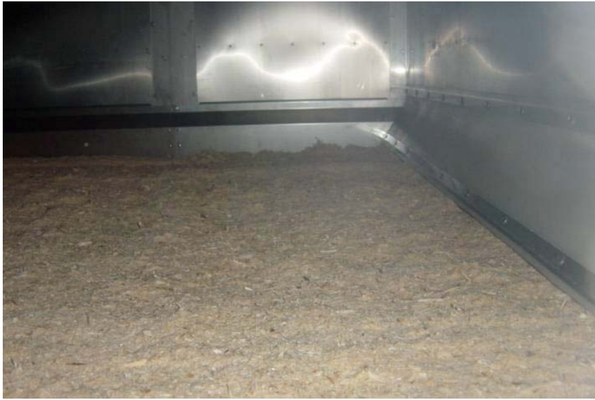
Fig. 6 Sawdust lying in a belt drier
